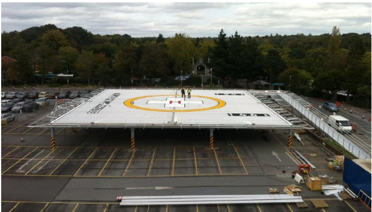
Figure 1: A heliport on a raised structure over a car park
